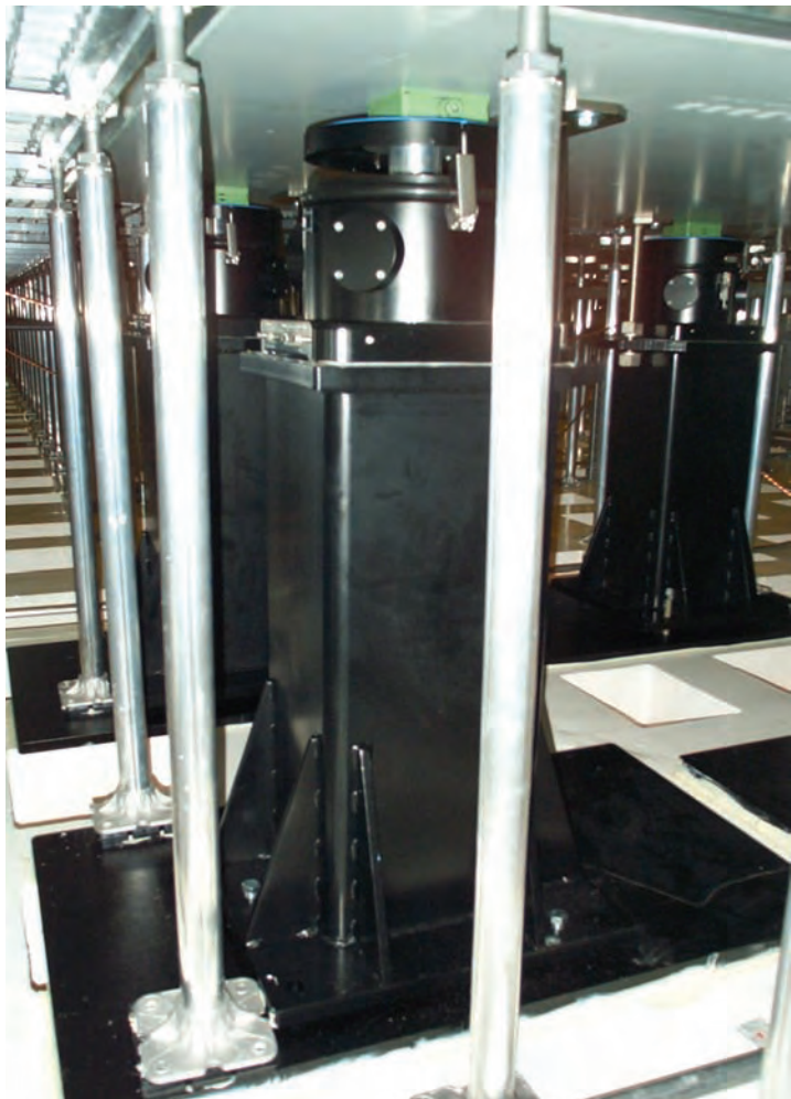
STACIS® 2100 on a "riser" installed under a TMC platform in a 40" tall raised floor
